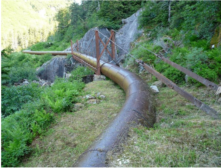
Figure 5-7. Upper Annex Lake Outlet, Penstock Bridge
