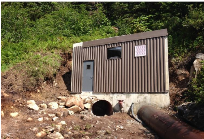
Figure 5-24. JUN-1100, Valvehouse (modern), located where JUN-1099, Tunnel Ends
