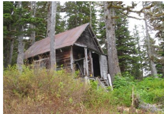
Figure 5-29. JUN-1111, Camp 4 Line Shack
