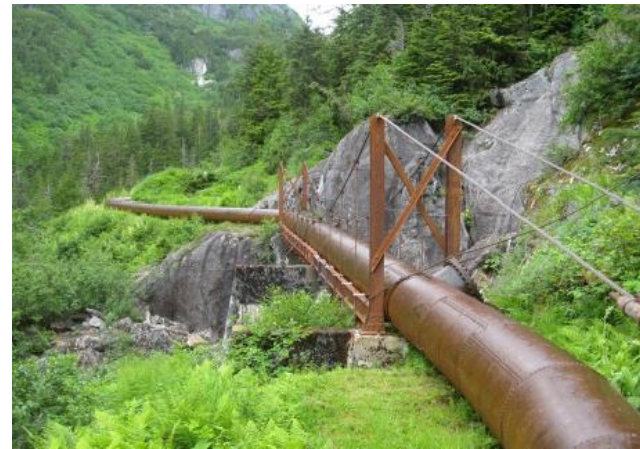
Figure 5-25. JUN-1101 and 1102, Penstock Pipeline and Bridge
