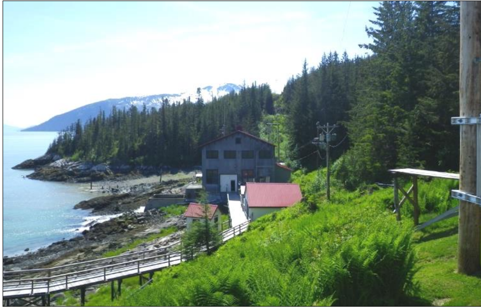
Figure 5-20. Annex Creek facilities
