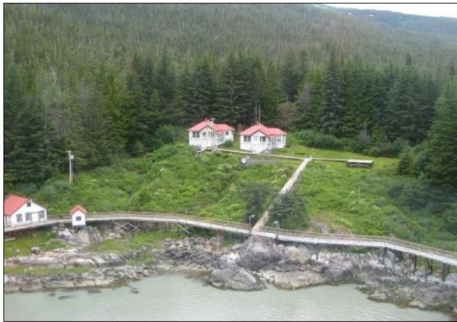
Figure 5-26. JUN-1103, Blacksmith/Carpentry Shop (far left); JUN-1104, Caretaker's House (rear right); JUN-1105, Employee's House (rear left)
