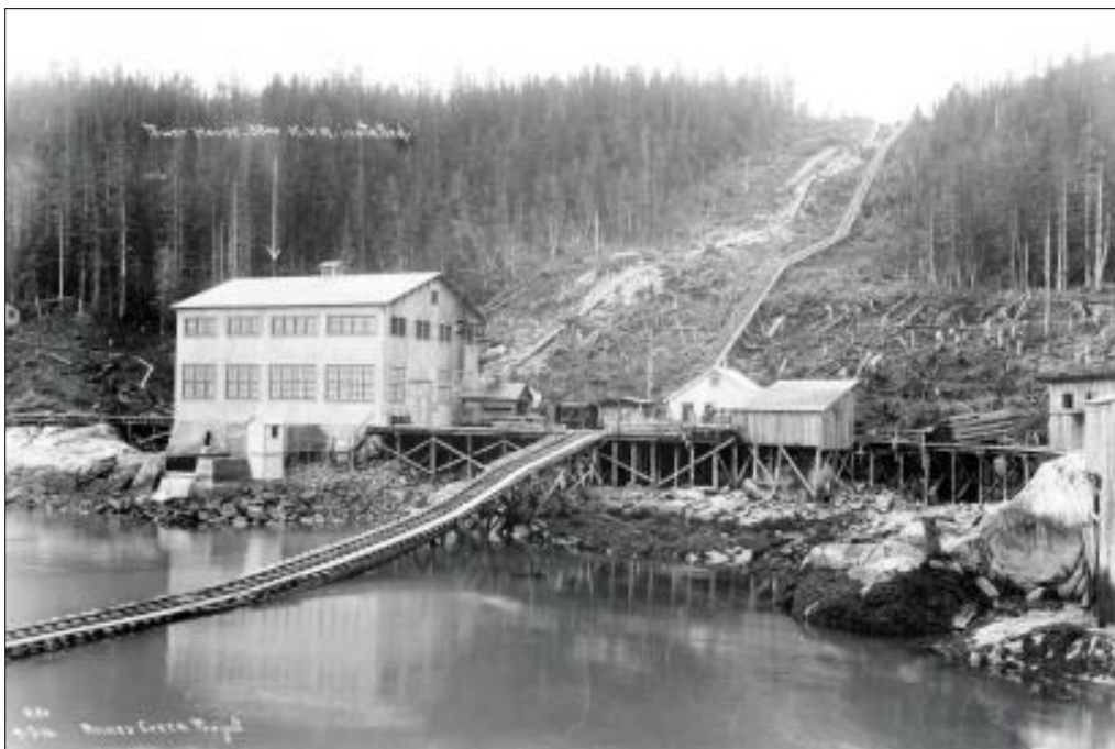
Figure 1-2. Annex Creek Powerhouse, 1916
