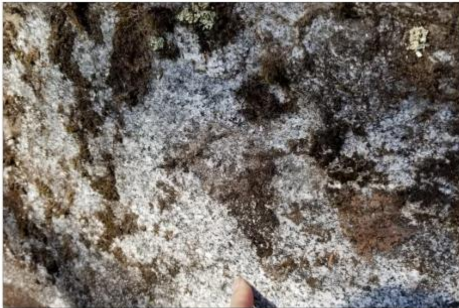
Figure 5-3. View of Typical Rock Observed along Penstock
