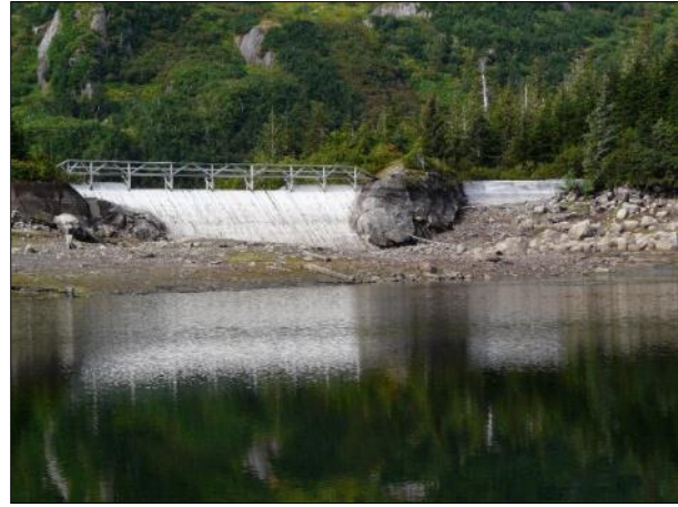
Upstream face of dam
