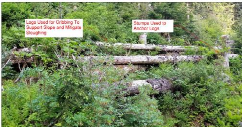
Figure 5-5. View of Timber Fallen near STA 30+50 to 31+25 (McMillen Jacobs 2019)
