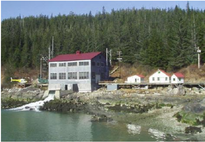
Figure 5-22. JUN-175, Hydroelectric Plant
