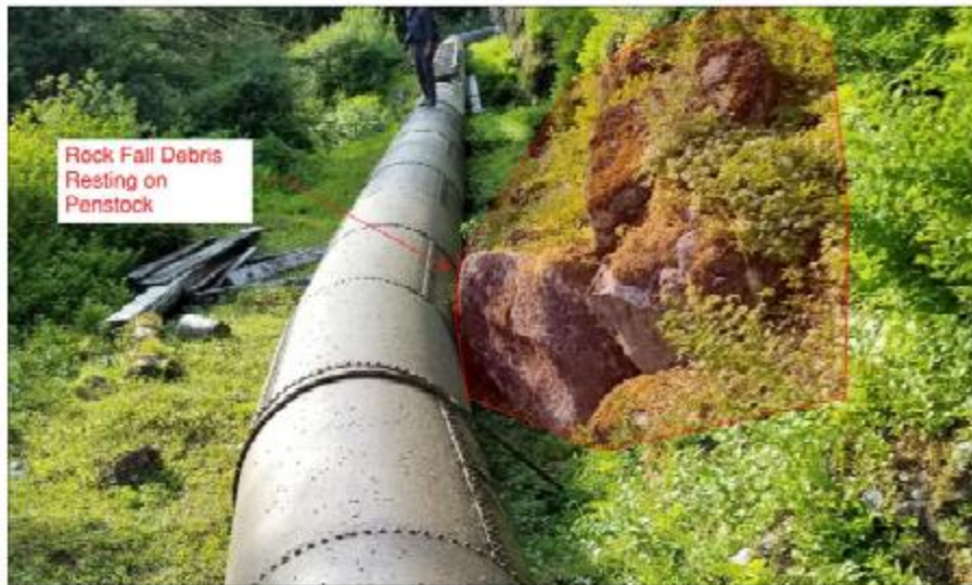
Figure 5-4. View of Rockfall Debris Observed near STA 26_75 to 27+50
