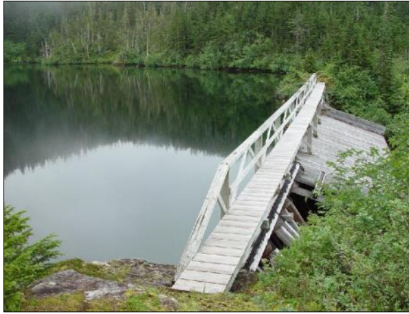
Dam and spillway
