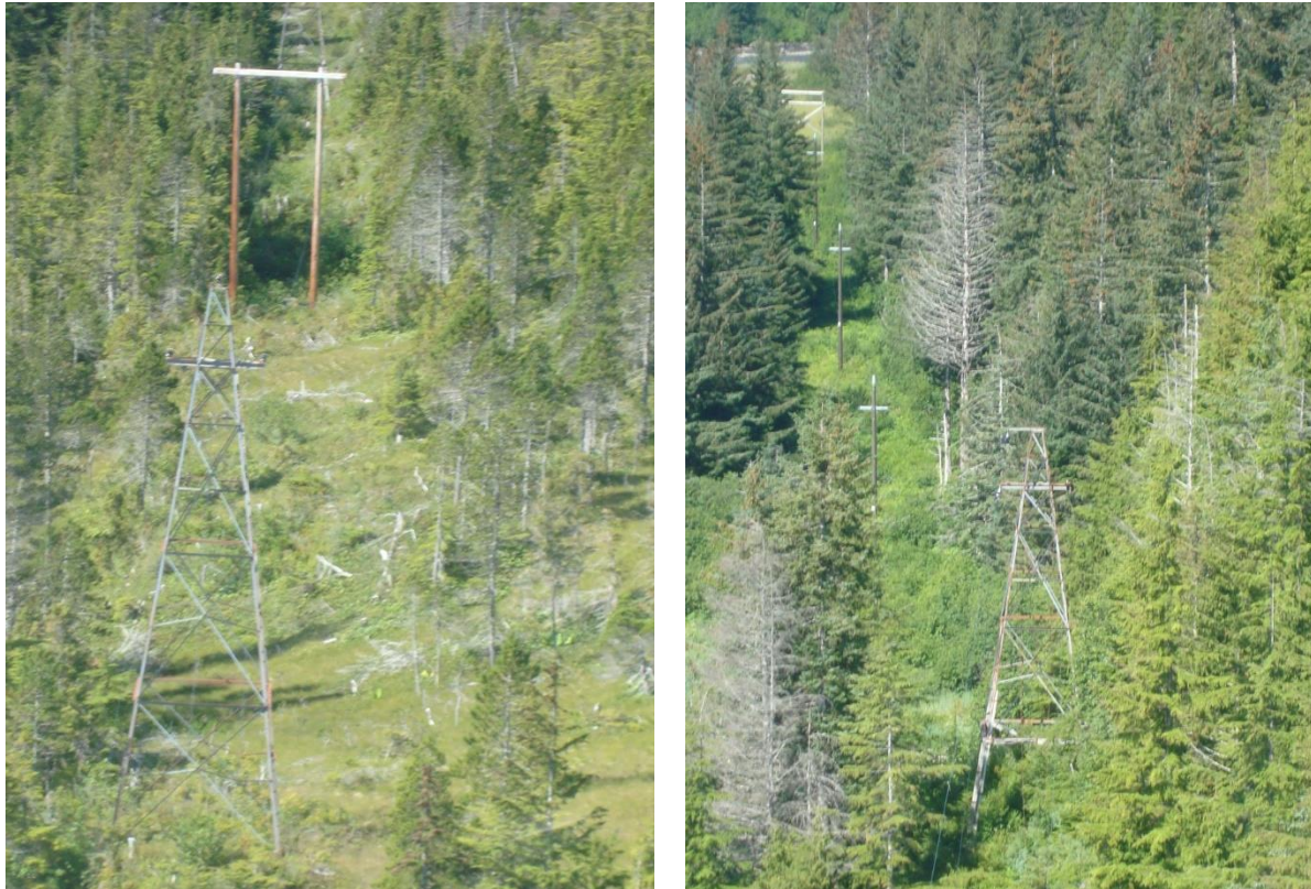
Figure 5-30. JUN-511, Power Line, showing towers prior to replacement
