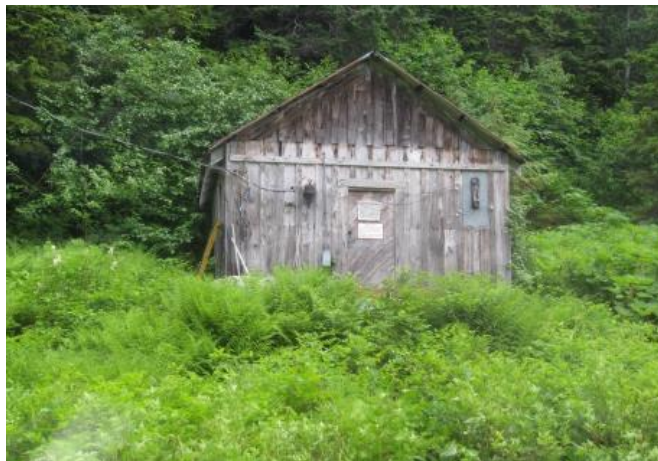
Figure 5-28. JUN-1110, Camp 2 Line Shack
