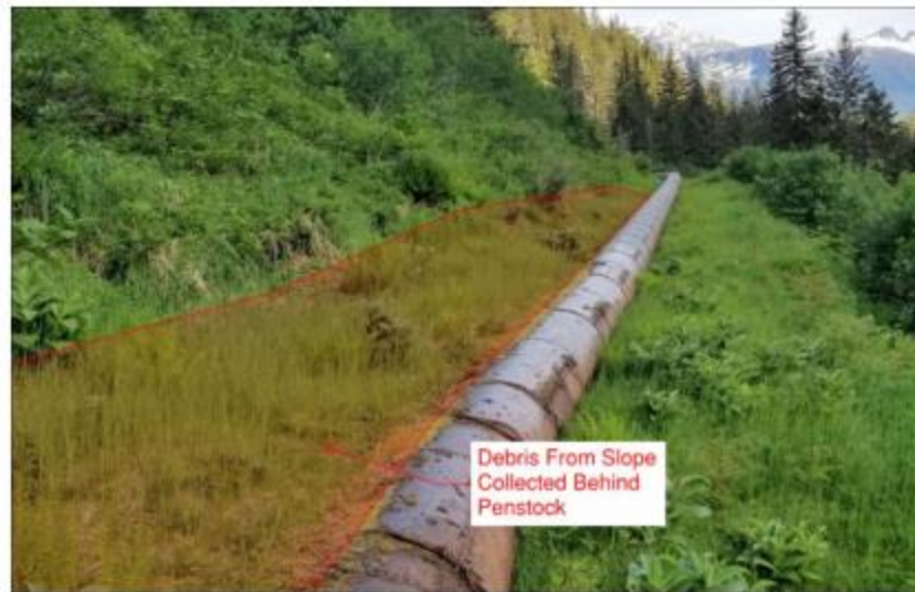
Figure 5-6. View of Sloughing Soil Accumulated behind the Penstock near STA 67+75 to 69+50
