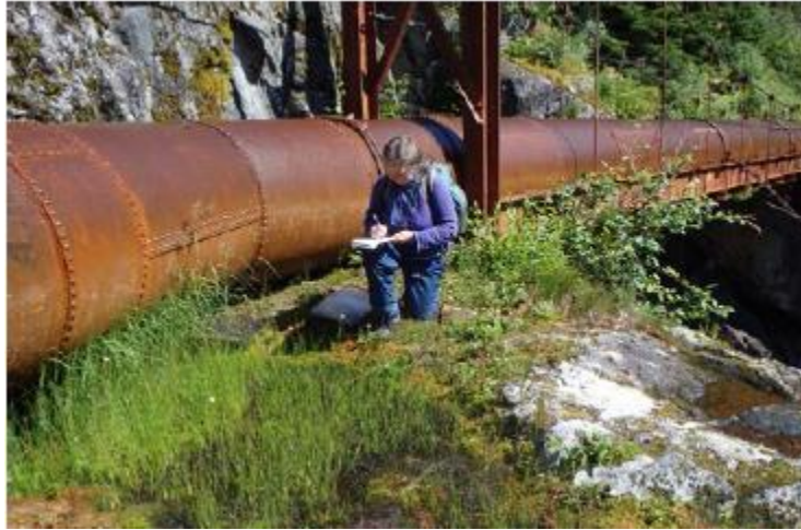
Figure 5-12. Survey along the penstock corridor
