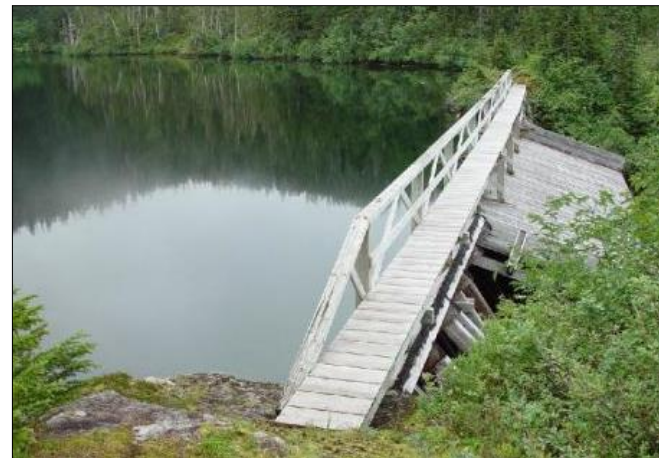
Figure 5-23. JUN-1098, Annex Creek Dam and Spillway
