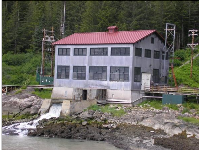
Figure 3-3. Annex Creek Powerhouse
