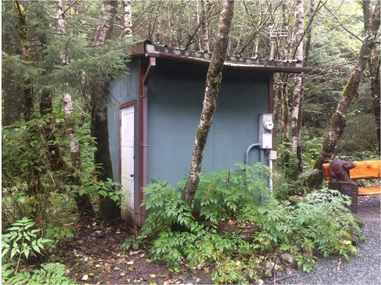
Figure 4. Showing the building housing the gage electronics located on the south bank just downstream of the pressure transducer.
