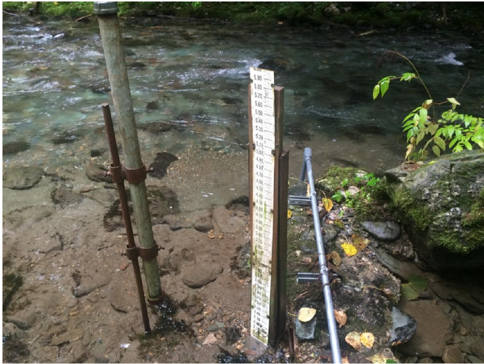
Figure 2. Showing USGS staff plate and orifice line containing the transducer.
